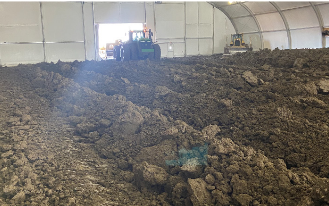
Warming tents were used to thaw the project's clay material during the last quarter of construction, Winter 2021.
