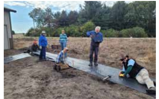
Laying the landscaping fabric below the walkway. Pictured (right to left): Marc Meijer, William Dittman, Phil Templeman, Joyce Dittman, Barb Meijer, Trevor Edmonson. © Alyssa Nyberg/TNC
