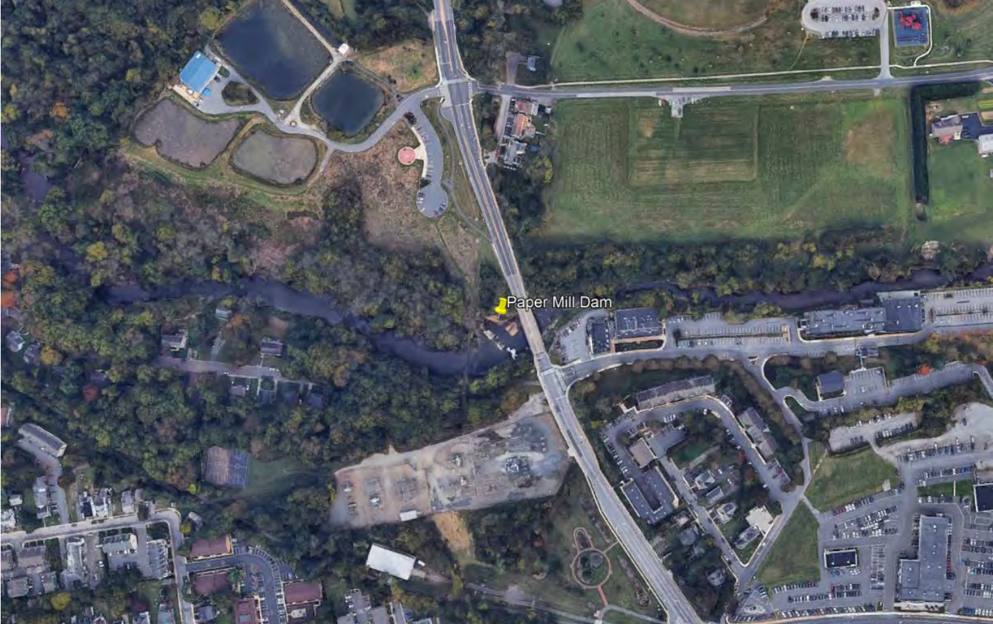
Paper Mill Dam aerial. Credit: Google Earth.
