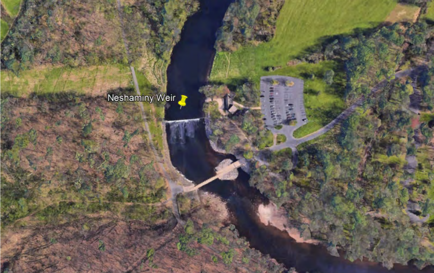
Neshaminy Weir Dam aerial. Credit: Google Earth.
