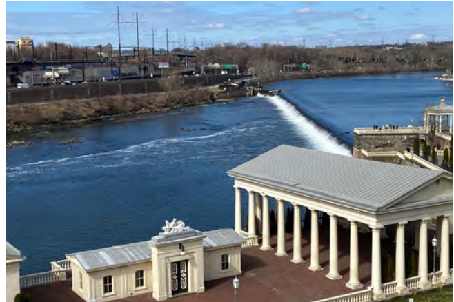
Fairmount Dam. Credit: Lyndon DeSalvo/TNC.
