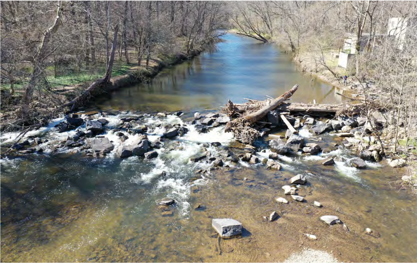
Deerfield Dam. Credit: Jason Fischel.
