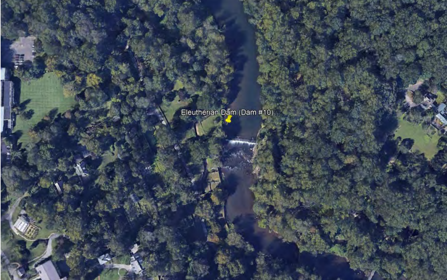
Eleutherian Dam aerial. Credit: Google Earth.
