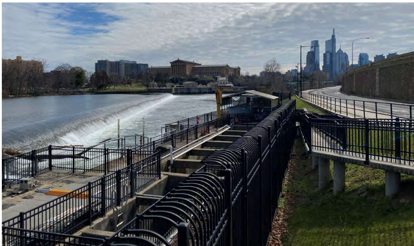
Figure 4-4. Fairmount Dam fish ladder. Credit: Lyndon DeSalvo/TNC.
