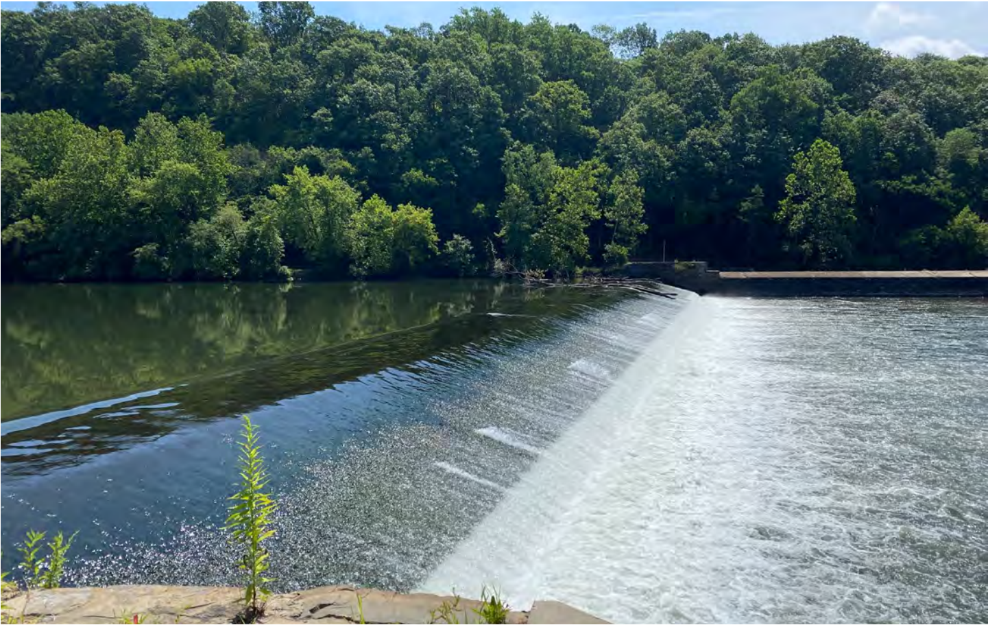
Black Rock Dam. Credit: Lyndon DeSalvo/TNC.
