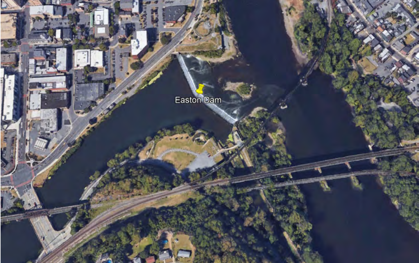
Easton Dam aerial. Credit: Google Earth.
