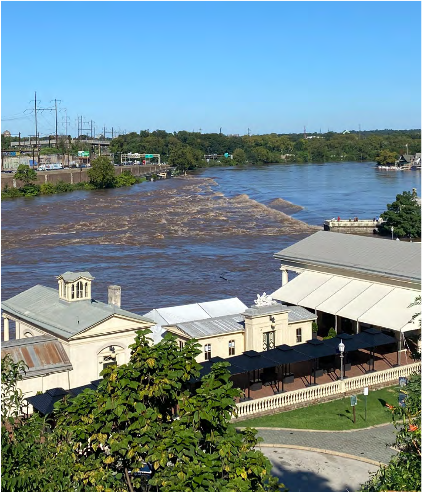
Figure 3-3. Fairmount Dam during Tropical Storm Ida, September 2021. The lower Schuylkill River severely flooded during Ida in September 2021 causing the Fairmount Dam to be completely submerged. During the storm, the fishway was damaged and may not be operational for the 2022 spawning runs. Credit: Lyndon DeSalvo/TNC.
