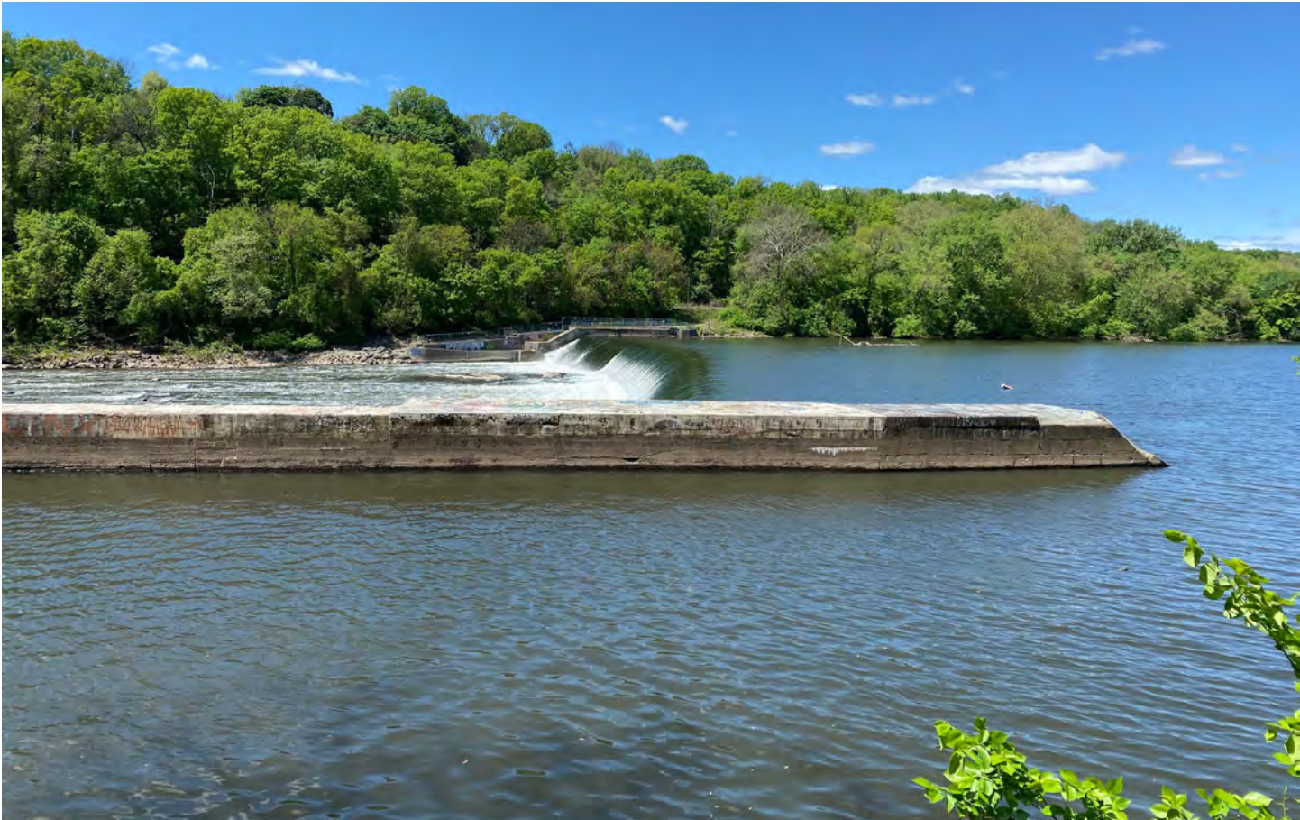
Flat Rock Dam. Credit: Lyndon DeSalvo/TNC.
