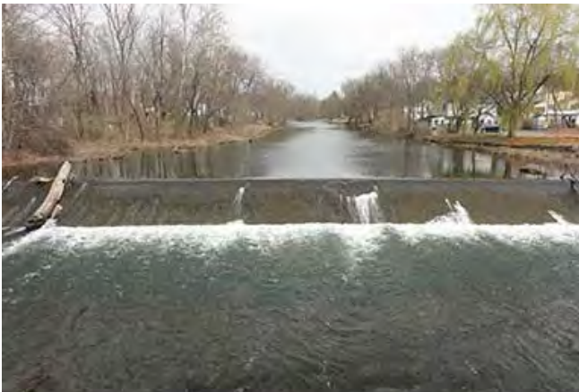
Bloomsbury Graphite Dam. Credit: NJ DEP.
