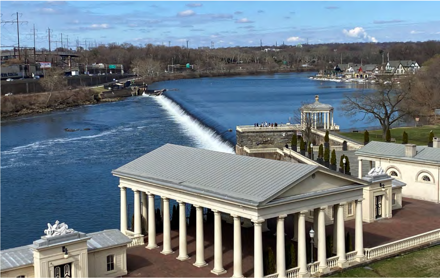
Fairmount Dam. Credit: Lyndon DeSalvo/TNC.
