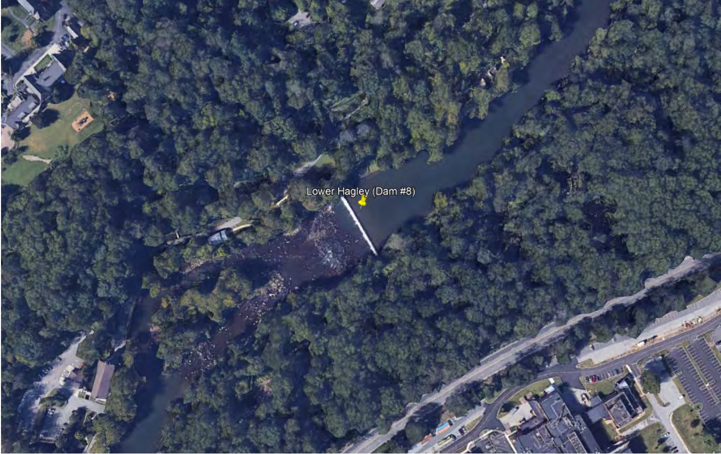
Lower Hagley Dam aerial. Credit: Google Earth.
