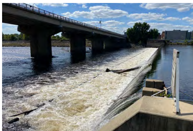
Hamilton Street Dam. Credit: Lyndon DeSalvo/TNC.
