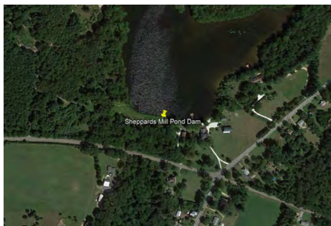
Sheppards Mill Pond Dam. Credit: Google Earth.
