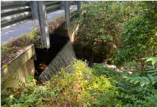
Clarks Pond Dam #2. Credit: Lyndon DeSalvo/TNC
