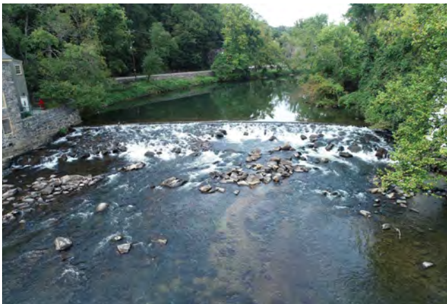
Breck's Mill/Walker's Mill Dam. Credit: Brandywine Shad 2020.
