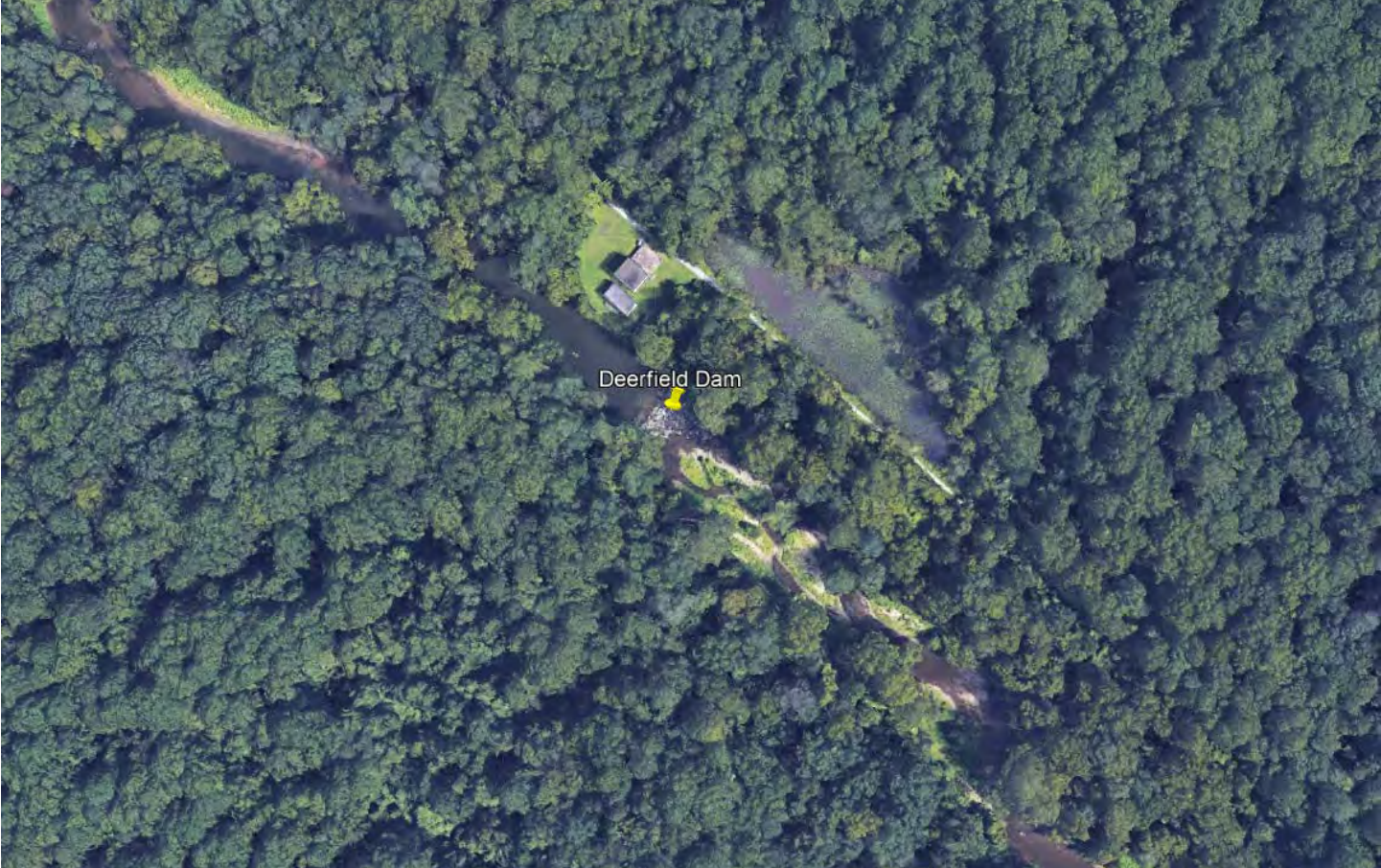
Deerfield Dam aerial. Credit: Google Earth.
