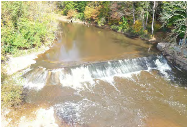
Newark Intake Dam. Credit: Jason Fischel.
