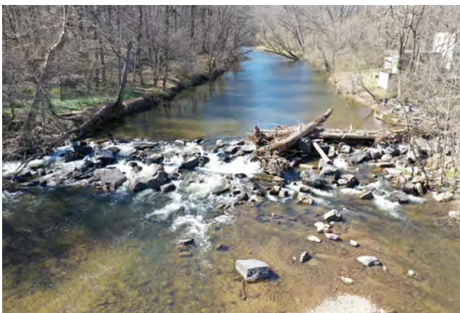
Deerfield Dam. Credit: Jason Fischel.
