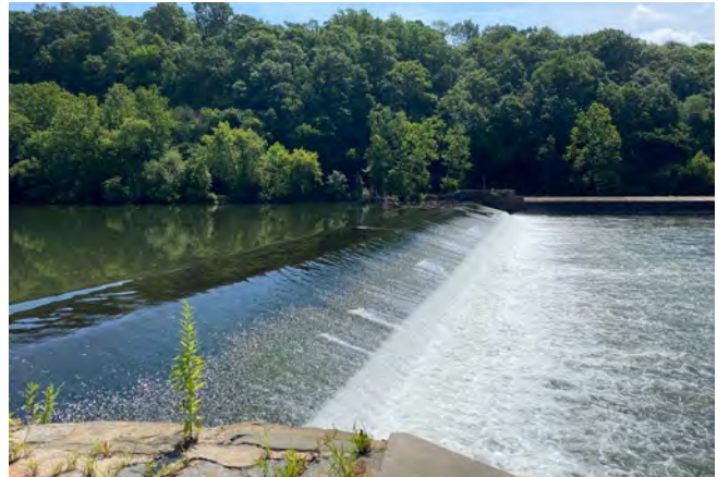
Black Rock Dam. Credit: Lyndon DeSalvo/TNC.
