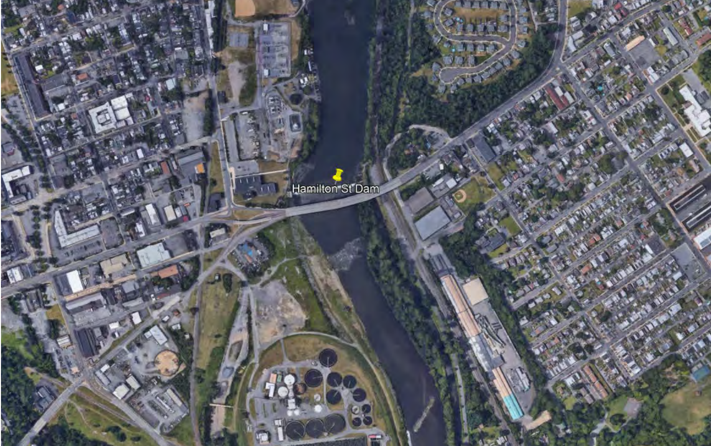
Hamilton Street Dam aerial. Credit: Google Earth.
