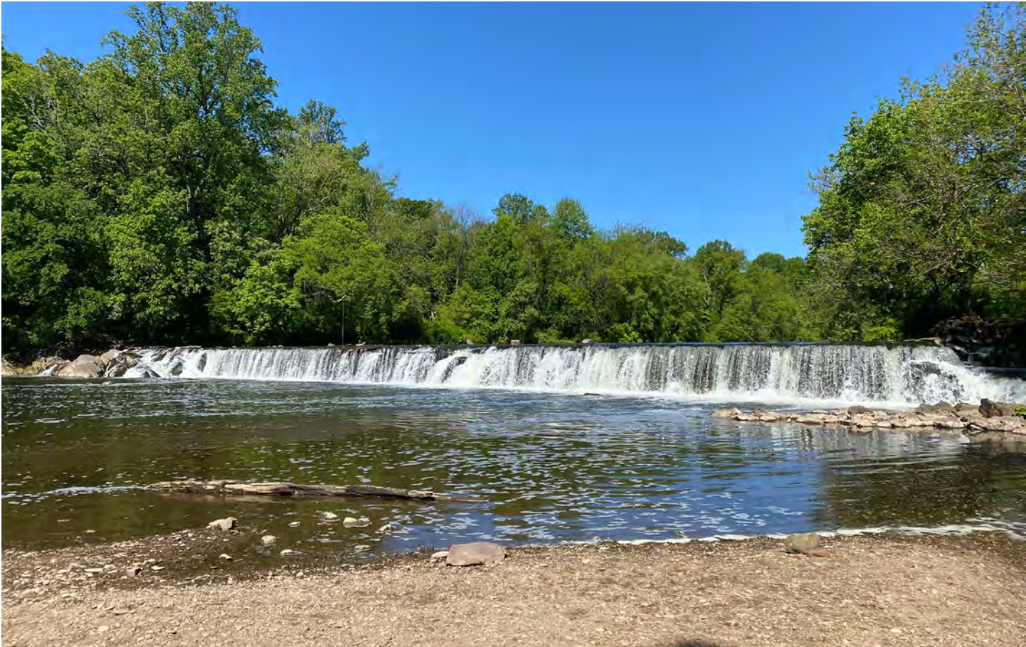
Hulmeville Park Dam. Credit: Lyndon DeSalvo/TNC.
