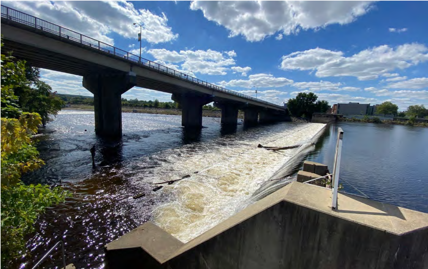
Hamilton Street Dam. Credit: Lyndon DeSalvo/TNC.
