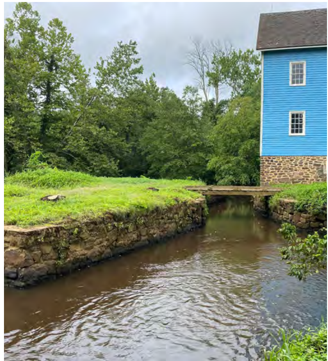
Figure 4-2. Walnford Dam on Crosswicks Creek. A side channel beside the historic gristmill was determined to allow for sufficient fish passage during a site visit. Credit: Lyndon DeSalvo/TNC.
