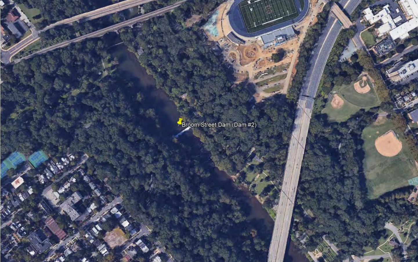
Dam aerial. Credit: Google Earth.
