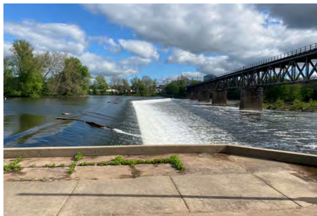
Norristown (Swede St) Dam. Credit: Lyndon DeSalvo/TNC.
