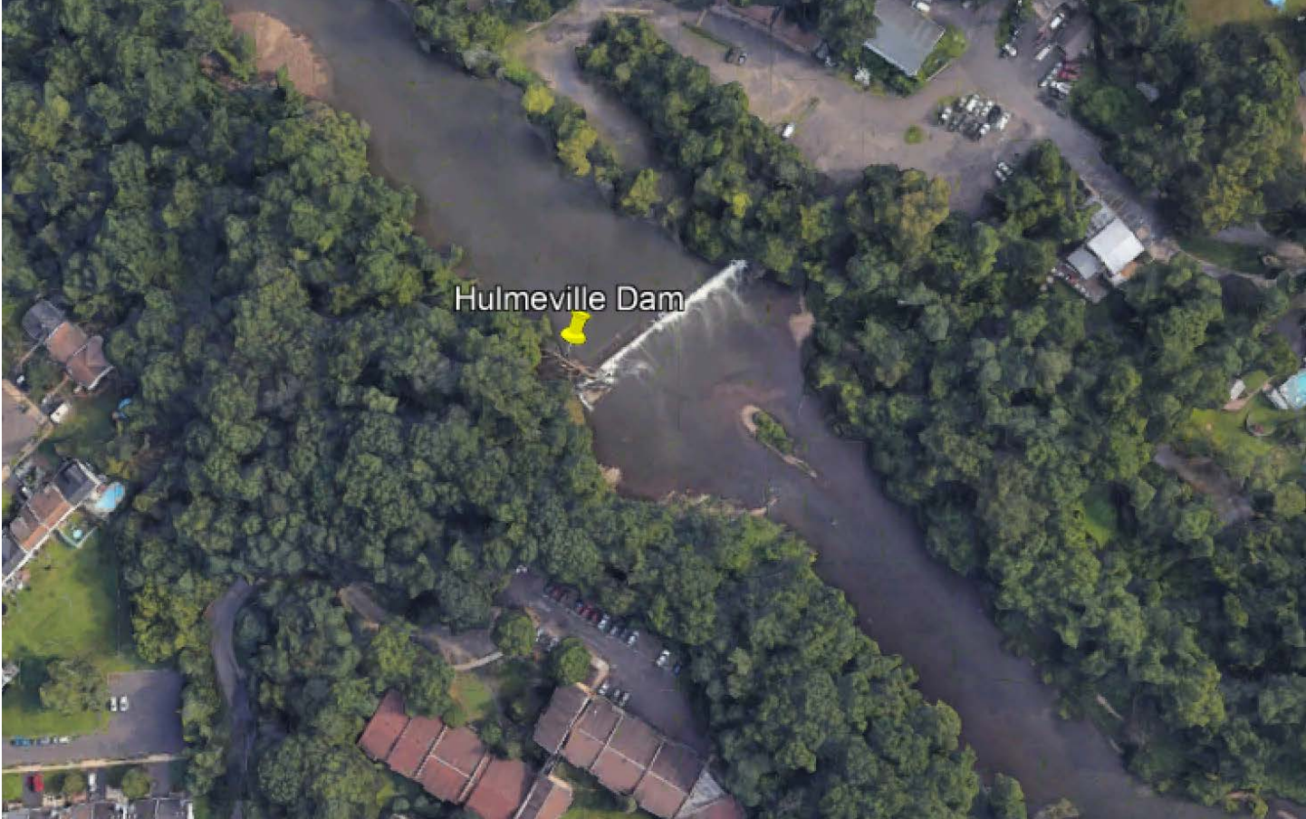
Hulmeville Park Dam aerial. Credit: Google Earth.
