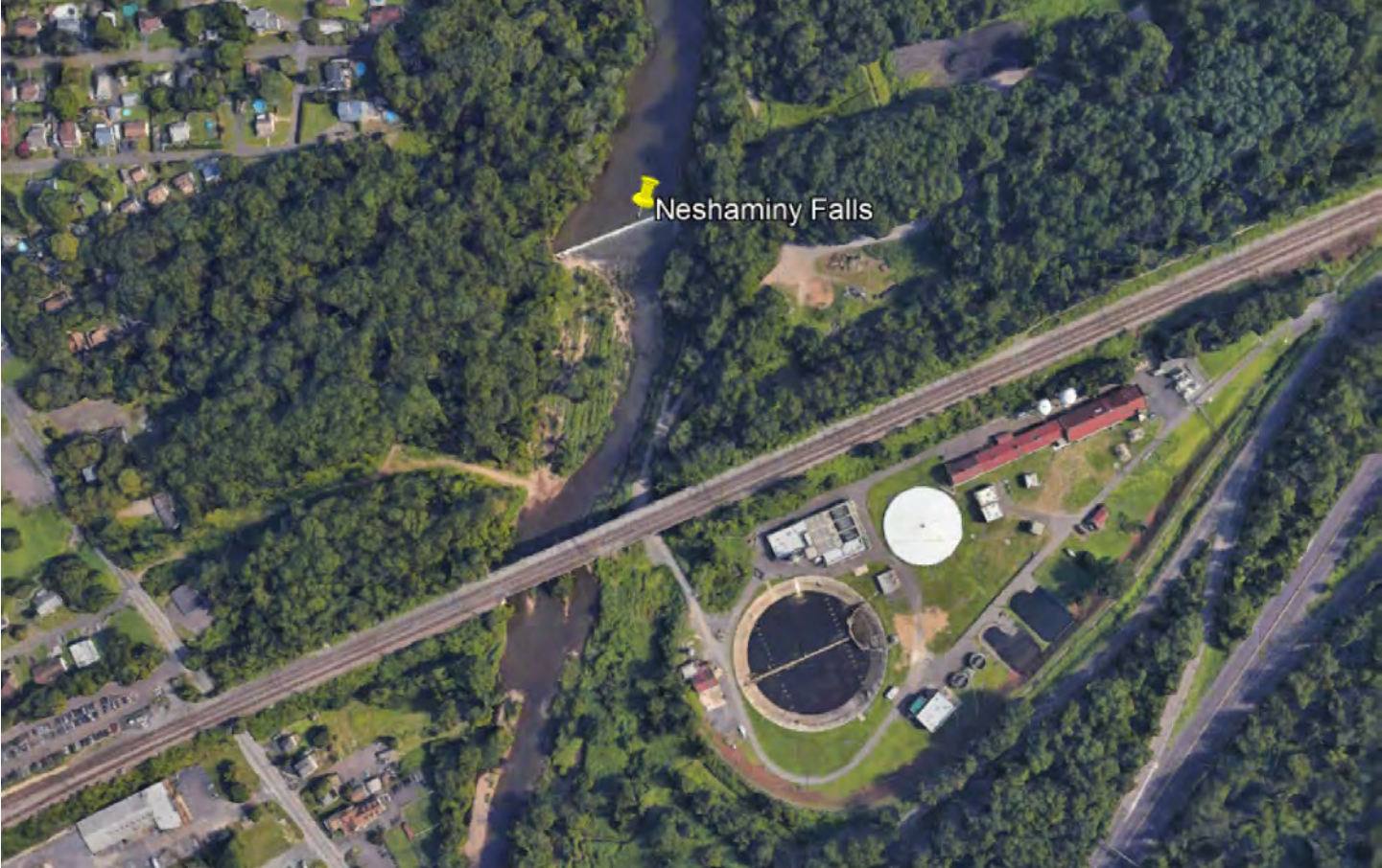
Neshaminy Falls Dam aerial. Credit: Google Earth.
