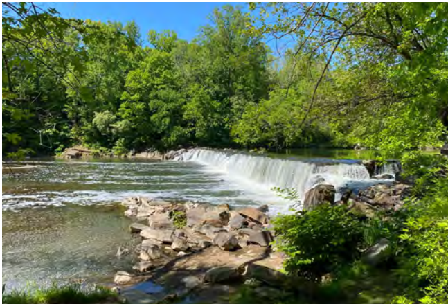
Hulmeville Park Dam. Credit: Lyndon DeSalvo/TNC.
