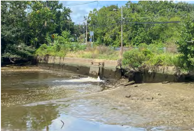
Clarks Pond Dam #1. Credit: Lyndon DeSalvo/TNC.
