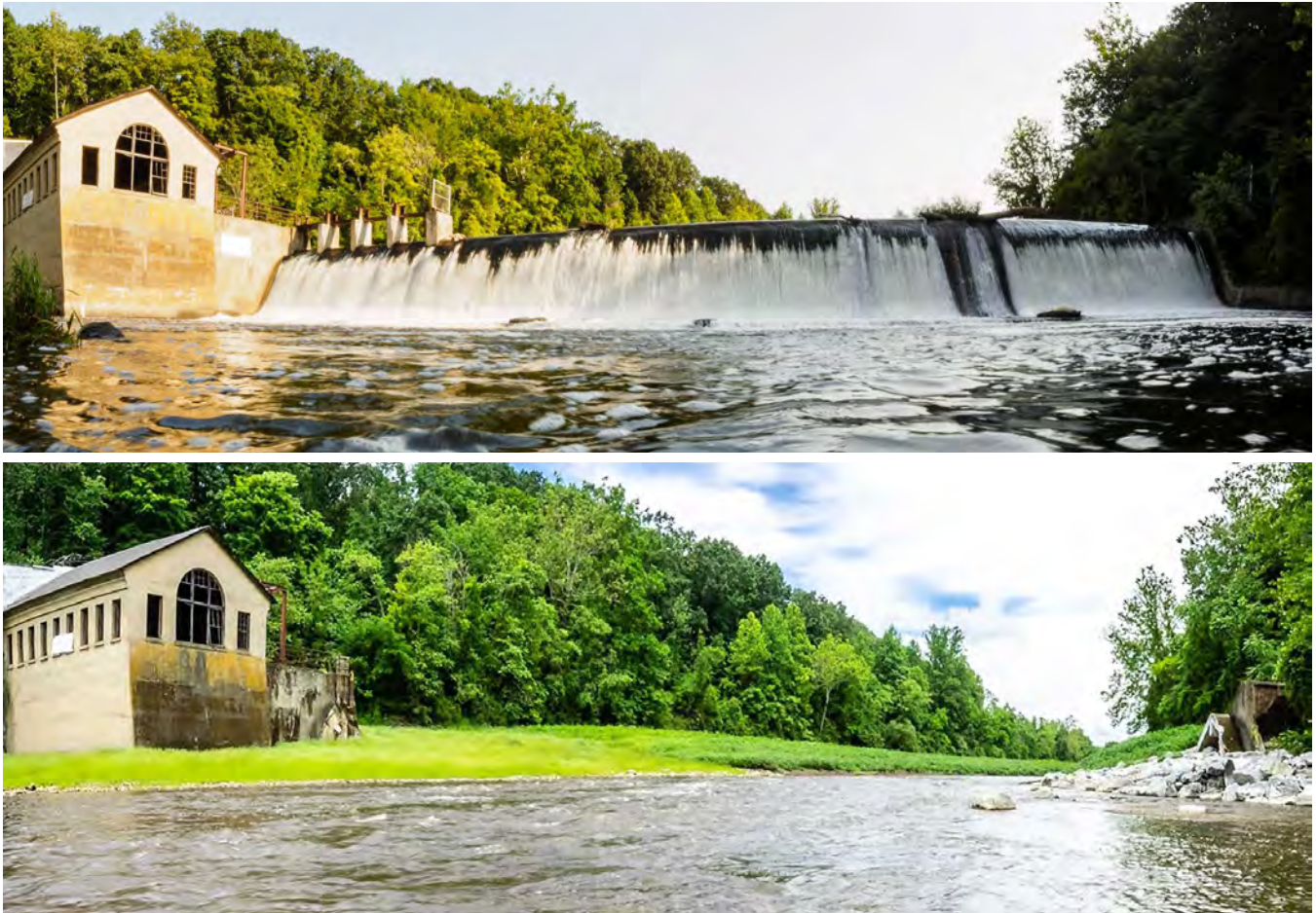
Figure ES-1. The Columbia Lake Dam on the Paulins Kill, before and after removal. Following the removal of the dam in 2018, American Shad and other migratory fish species now have access to an additional 10 miles of habitat upstream of the former dam site. Credit: Jeffrey Burian/TNC.
