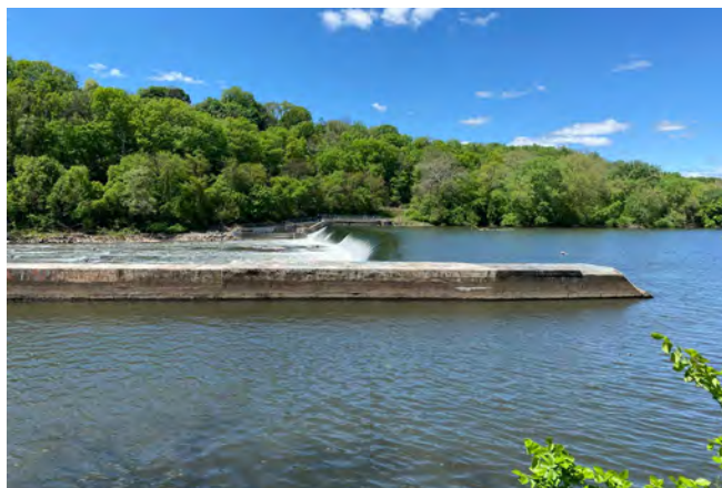
Flat Rock Dam. Credit: Lyndon DeSalvo/TNC.
